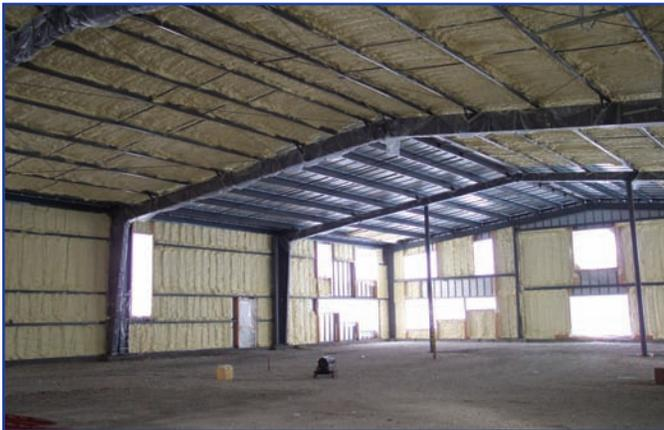
*Icynene soft foam insulation was sprayed at an average depth of 4-5 inches onto steel wall panels, gable ends and the underside of the steel roof.*
