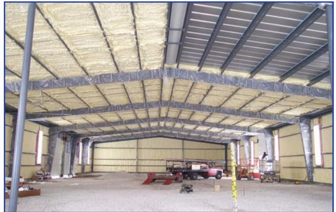
*Once Icynene was applied to the steel wall panels, tests revealed that the PFI building achieved an airtightness level better than that of a tight residential structure.*
