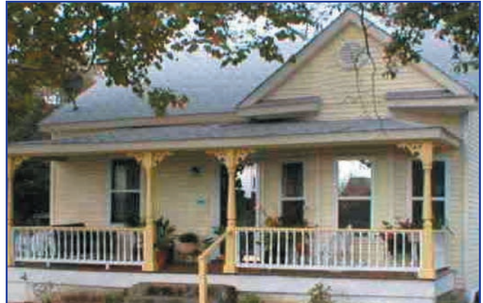
Icynene was key in restoring this heritage home, which was once considered irreparable. Now, the home provides the owner with a Healthier, Quieter, More Energy Efficient® environment.
