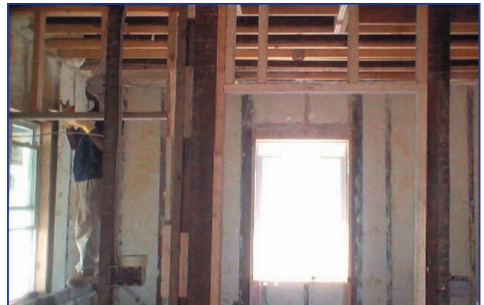
Icynene is water-blown and does not contain synthetic blowing agents such as HFCs. An Icynene-insulated environment is highly recommended for those suffering from allergies, respiratory problems and chemical sensitivities.
