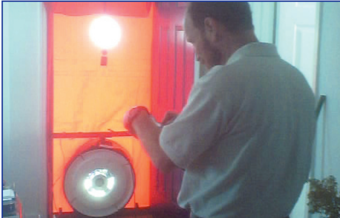
After the Icynene® application, blower door test data confirmed that this home met and exceeded the energy efficient requirements for designation as an EPA Energy Star® Home.
