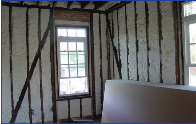
The air tight building envelope construction allows for optimum heating and cooling cycles and reduced energy costs.
