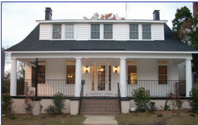
The new HBA office building got a complete facelift inside and out while heating bills were reduced by a remarkable 92%.
