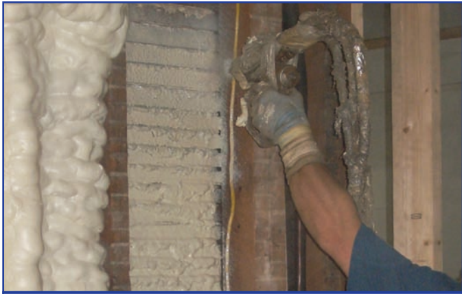
When sprayed, Icnene expands 100 times and completely adheres to the substrate reducing the chances of any air gaps forming inside the wall cavity.
