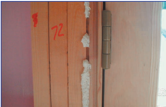
Icnene softly expands to 100 times its initial volume to completely fill all gaps and crevices that compromise airtightness.
