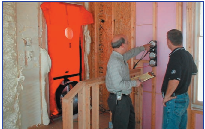
A blower door test was conducted to measure airflow, which proved that the most significant reduction in airflow was the result of the Icnene application alone.
